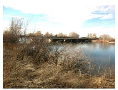
the FEMA predicted 100-year water elevations approximately 0.5 feet under the low chord of the bridge, including the FEMA estimated effects of ice jams.
